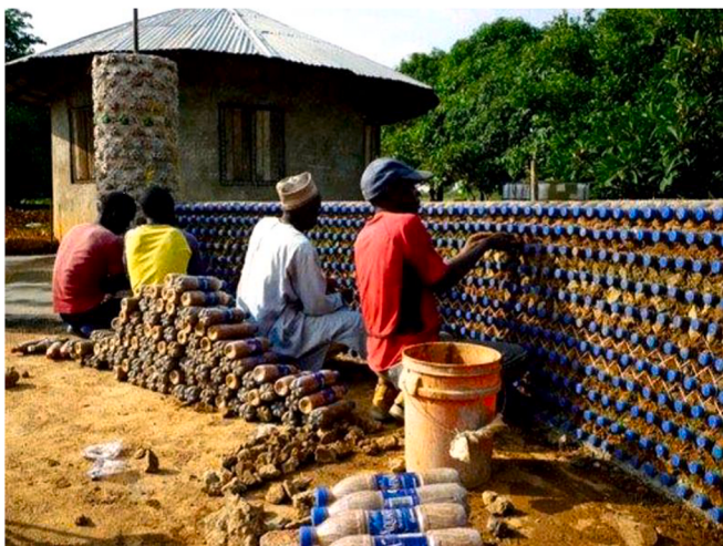
Fig. 10. Local people constructing their own living shelters by utilizing waste plastic bottle as plastic brick in Nevada (Haque, 2019).
